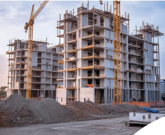
Tower crane-provides emergency power
