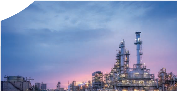
Industrial site-independent power supply
