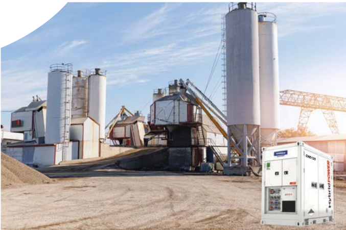
Small-scale factory-provides independent power
